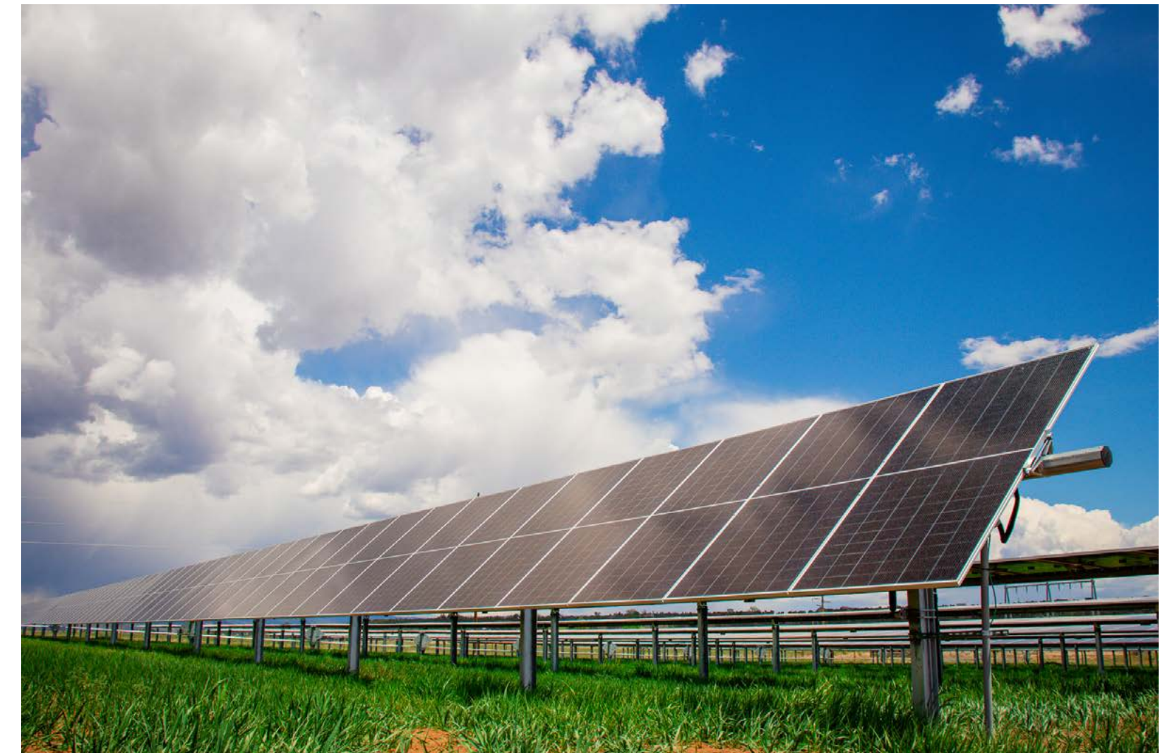
Progress continued at Sunnyside Community Solar.
