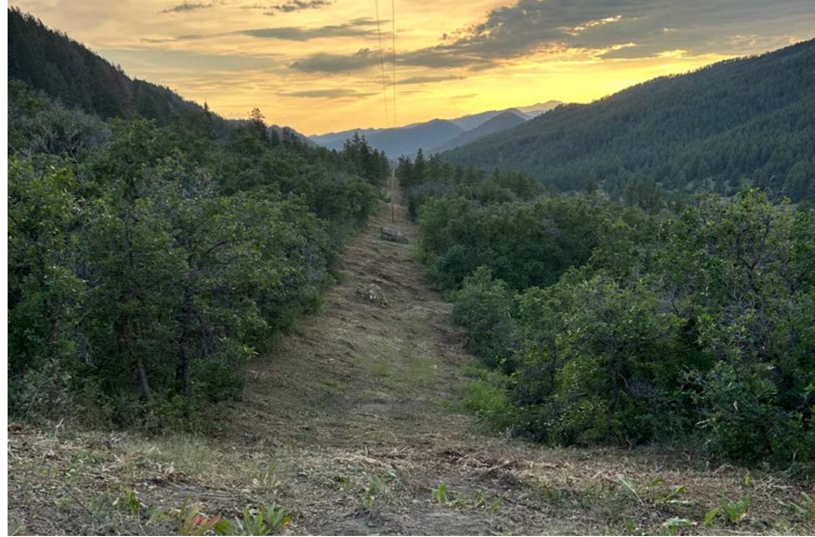
Vegetation clearing on the Bear Creek to Pine Springs Line.
