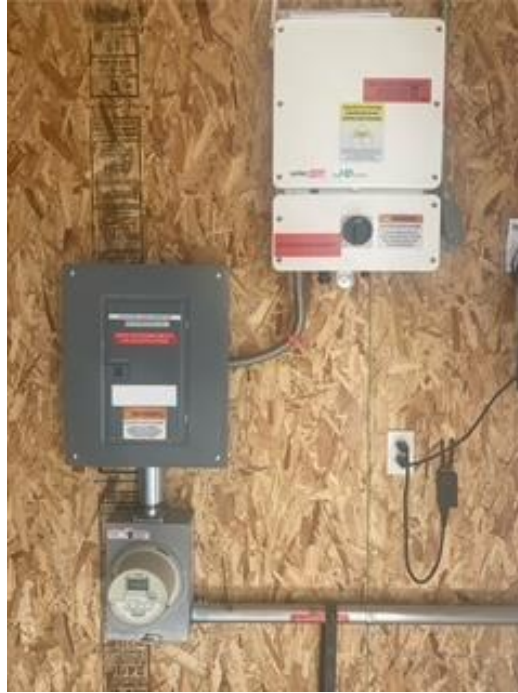
Labeled AC Disconnect
