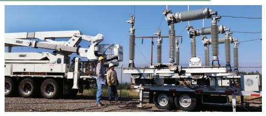
Performing routine maintenance and necessary repairs on any of LPEA's 30 substations is made much easier thanks to one piece of equipment in LPEA's arsenal: our mobile substation. It allows our crews to de-energize critical electrical infrastructure without causing outages and is regularly used across LPEA's service territory to fix and replace aging equipment.
