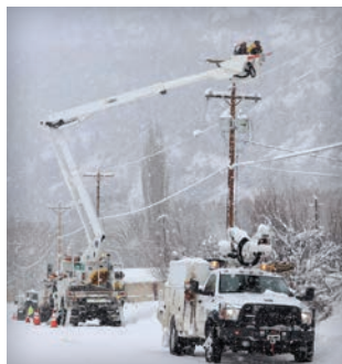
Restoring power during the February 2019 snowstorm.
