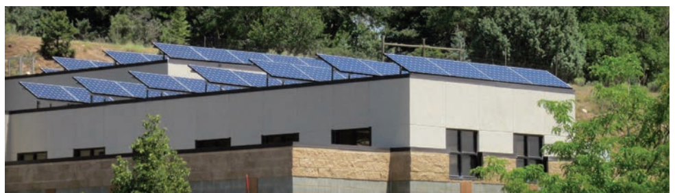
Solar installation in LPEA service area.
