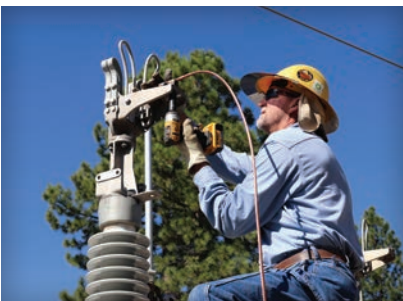
Steve Lynch upgrades equipment at LPEA substation.
